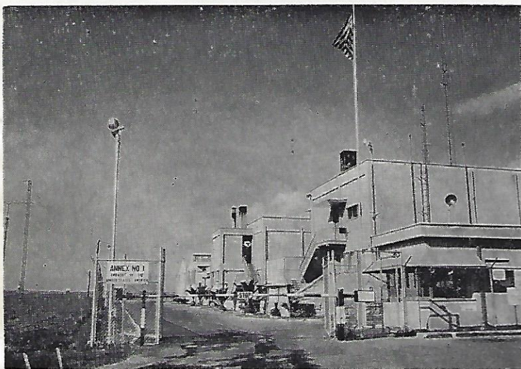
RADIO RELAY STATION
