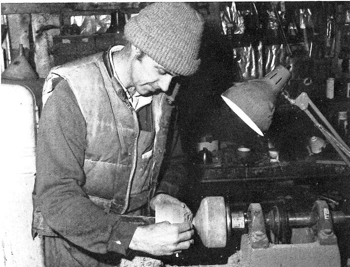
Dick Fischer begins processing the bells by shaping wooden forms on a lathe.
